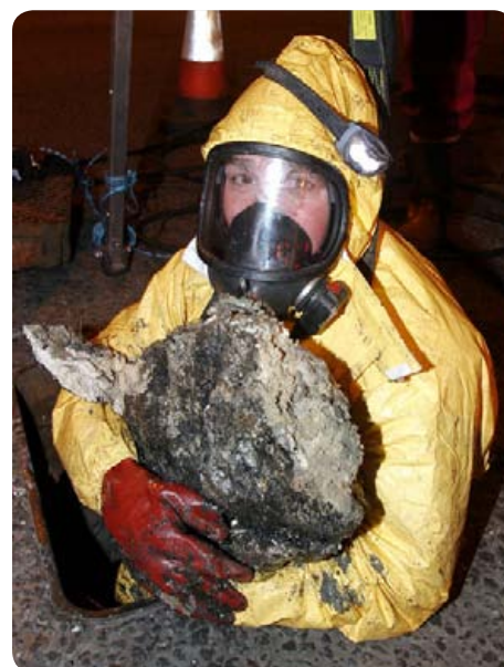
A Thames Water engineer emerging from a sewer with a lump of 'fatberg'
